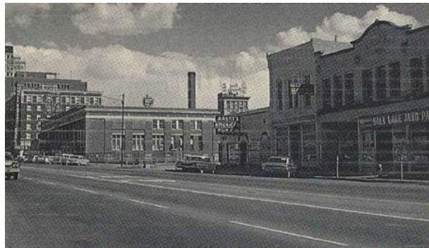
View before excavation for Salt Lake Auto Parts Utah Nippo Long Hotel American Fur Co and the Greyhound Bus Depot
