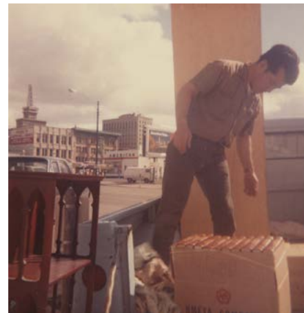
Moving supplies out of the Aloha Cafe before its demolition
