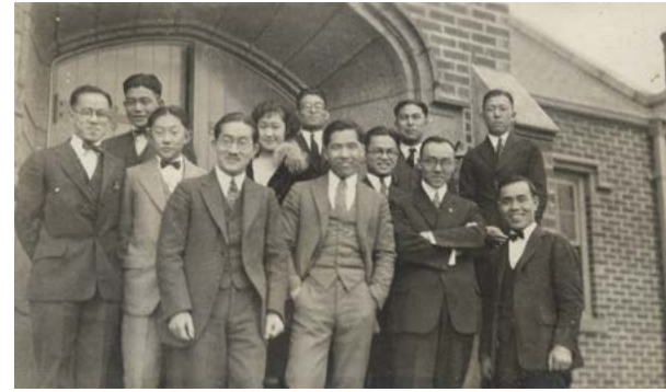
Group of men on the front steps of the newly constructed church
