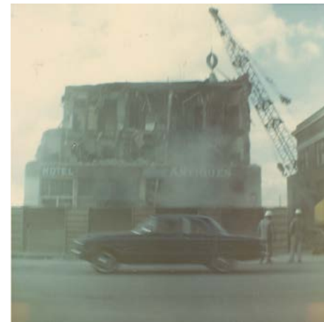
Demolition of Japantown making room for the new convention center
