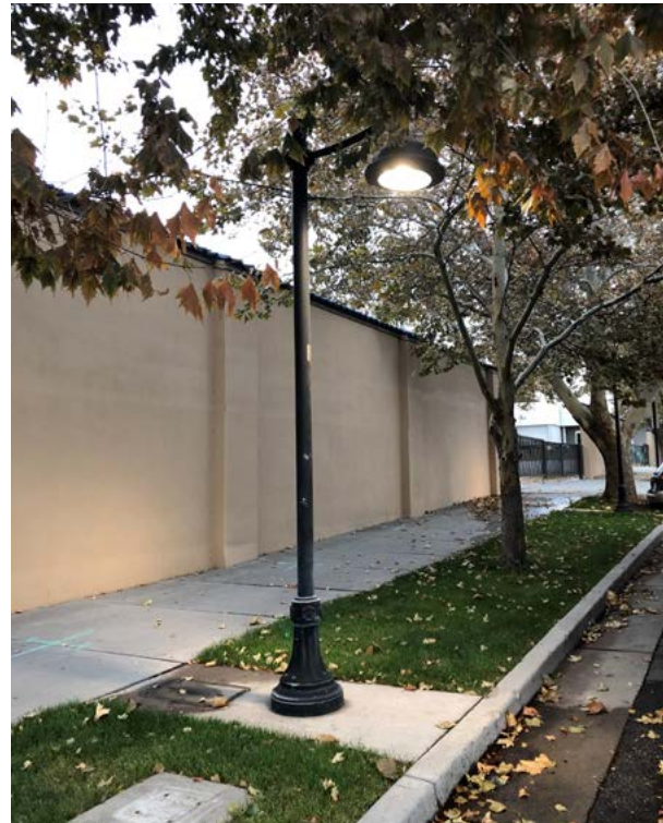
North side of Japantown Street, 3 specialty pedestrian pole ("lantern" style)
