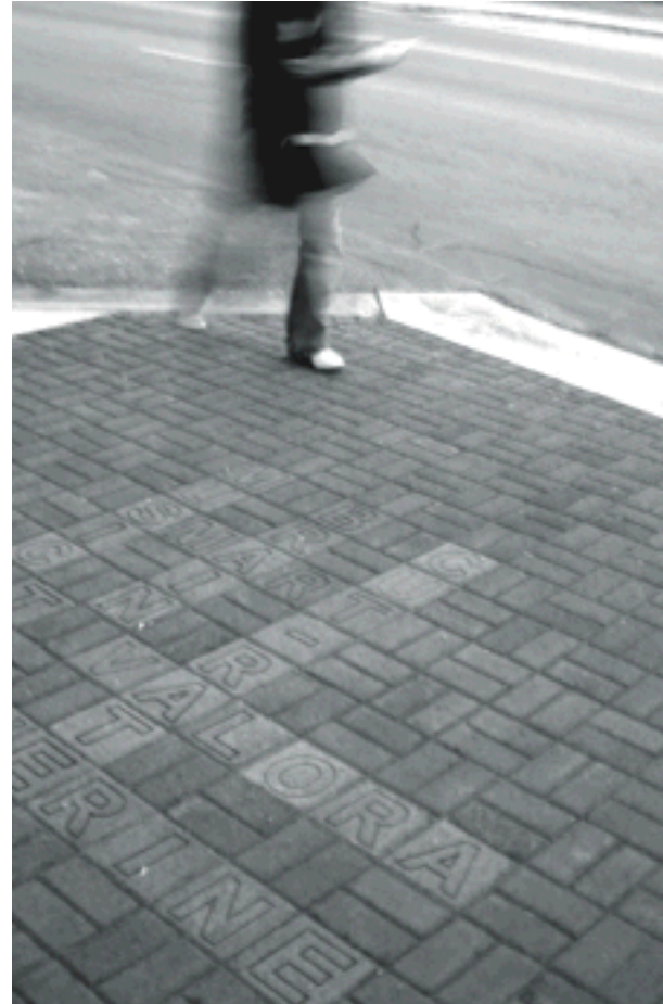
The Paver Replacement Project in the Sugar House Project Area
