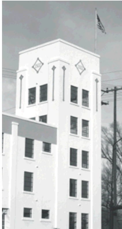
Big D Construction's renovated Fuller Paint Building
