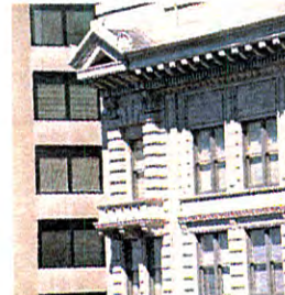
Clift Building detail
